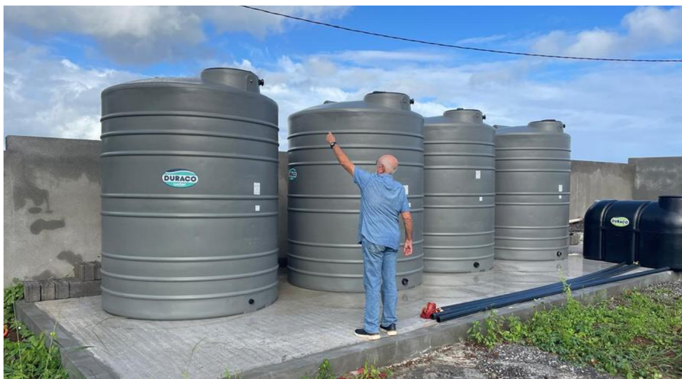
The 4 water tanks of 9000L installed on the newly built concrete slab.
